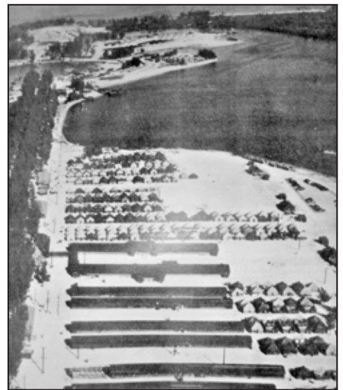
This aerial photo shows the main layout of the base including barracks, tents and training sites south of the inlet. Outlying facilities were along both north and south beaches where access was restricted. U.S. Navy photo.
